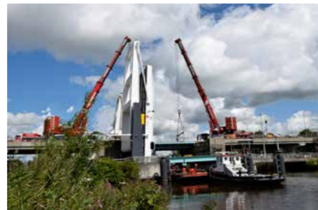
April: Lifting the Euvelgunner bridge
