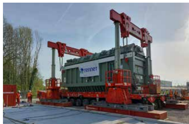
May: Transformers in transport
